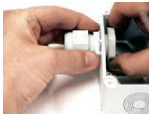
Install the cable glands.
