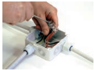
Insert the cables and connect the wires.
