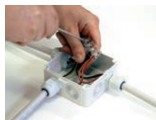
Insert the cables and connect the wires.
