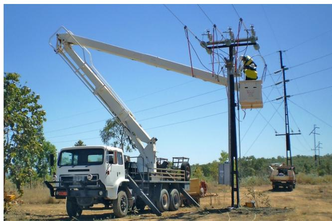
OSM Recloser installation to reduce maintenance costs and lost production time at GBS Mine
